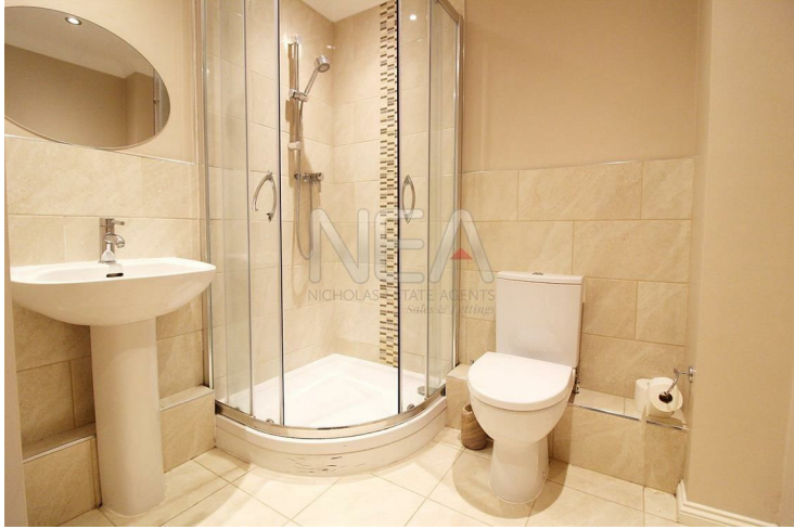
Cubicle shower, sink, WC, cupboard housing hot water tank
